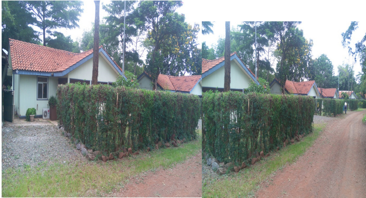
Activities on progress at Orka village early stage
