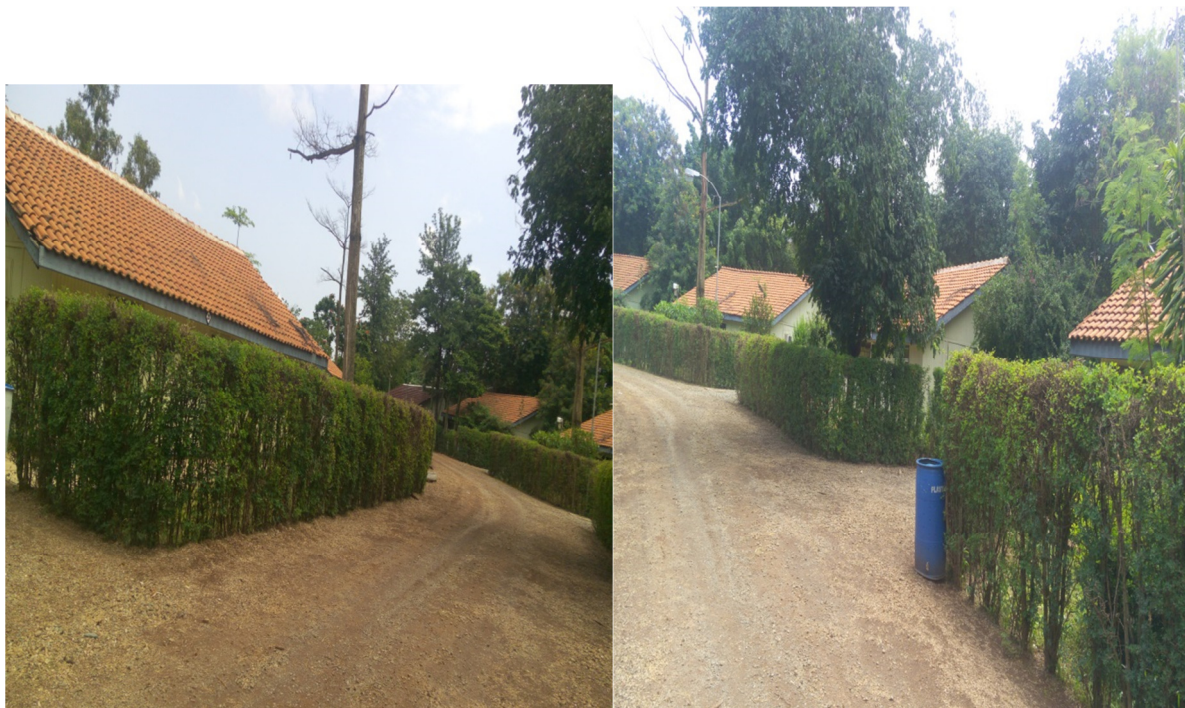
Finishing stage at Orka village.
